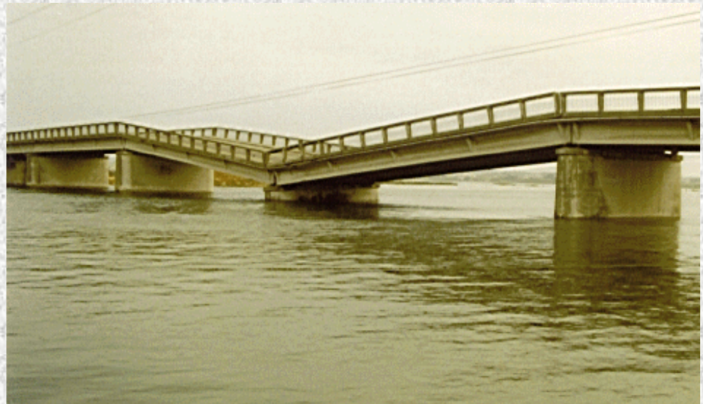
Gafanha bridge in Aveiro
